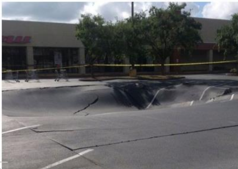
The parking lot at a Publix near Legoland in Winterhaven is buckling and dipping due to a suspected
