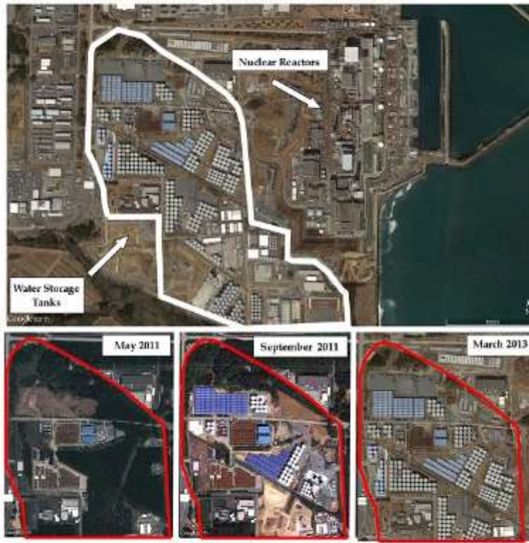
Growth of Water Storage Tank Farm at the Fukushima Daiichi Nuclear Power Station
