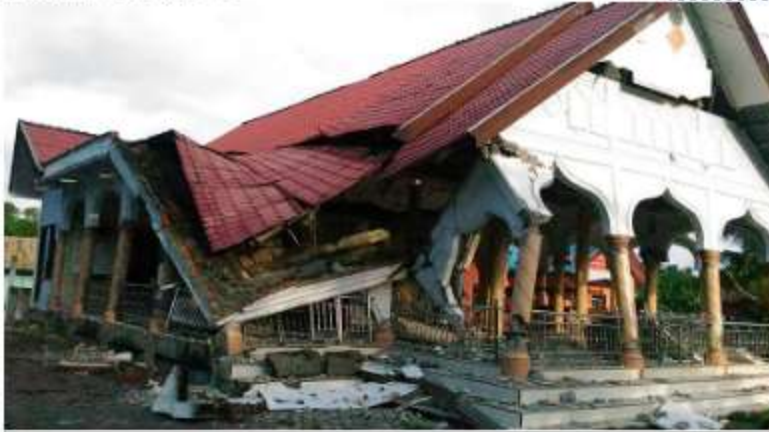
A badly damaged building is seen after a 6.5-magnitude earthquake struck the town of Pidie, Indonesia's Aceh province in northern Sumatra, on December 7, 2016 © Zian Muttaqien / AFP
