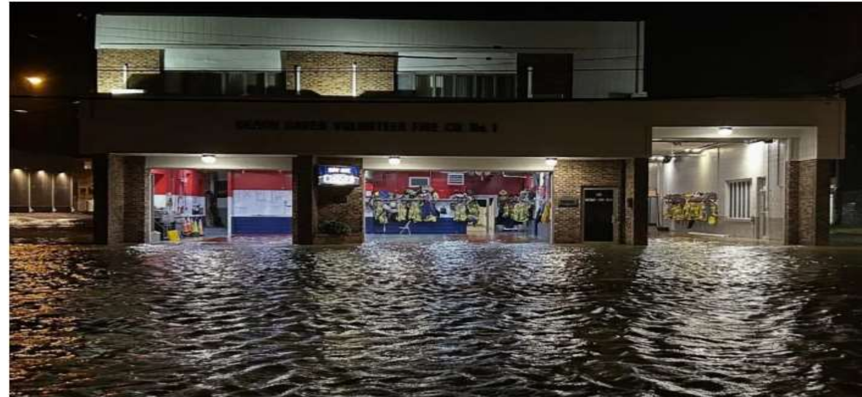
Floodwaters breach the Beach Haven Volunteer Fire Department on October 13, 2025. Credit: Beach Haven Volunteer Fire Department
