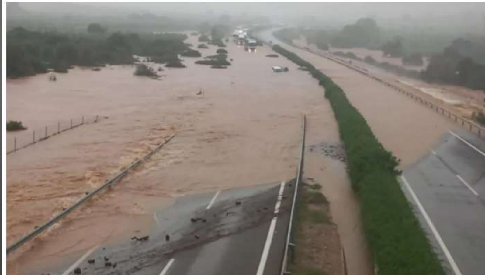
Flooded AP7 motorway in Spain on October 11, 2025. Credit Meteocat
